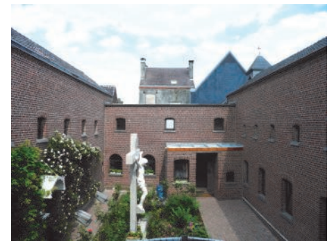
The inner courtyard of the Carmel du Sacre Coeur, Quievrain, Belgium.
