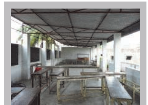
St. Anthony's Chapel (see opposite page, far left) was built on the roof of St. Anthony's School. This is what it looked like before construction started.
